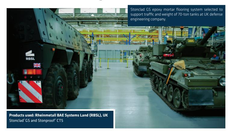
Single-source industrial flooring specialist Stonhard has met one of its heaviest challenges in years by laying a high-performance, power-troweled epoxy mortar floor to withstand traffic from 70-ton tanks manufactured by a UK-based defense engineering company.
