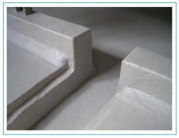
Stonchem glass fibre reinforcing membrane installed to all areas to provide strategic strengthening to the lining system.
